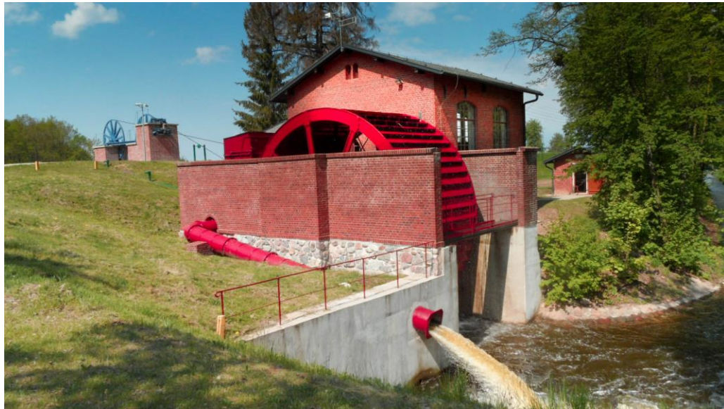
Photo 10. The machine room with the waterwheel
